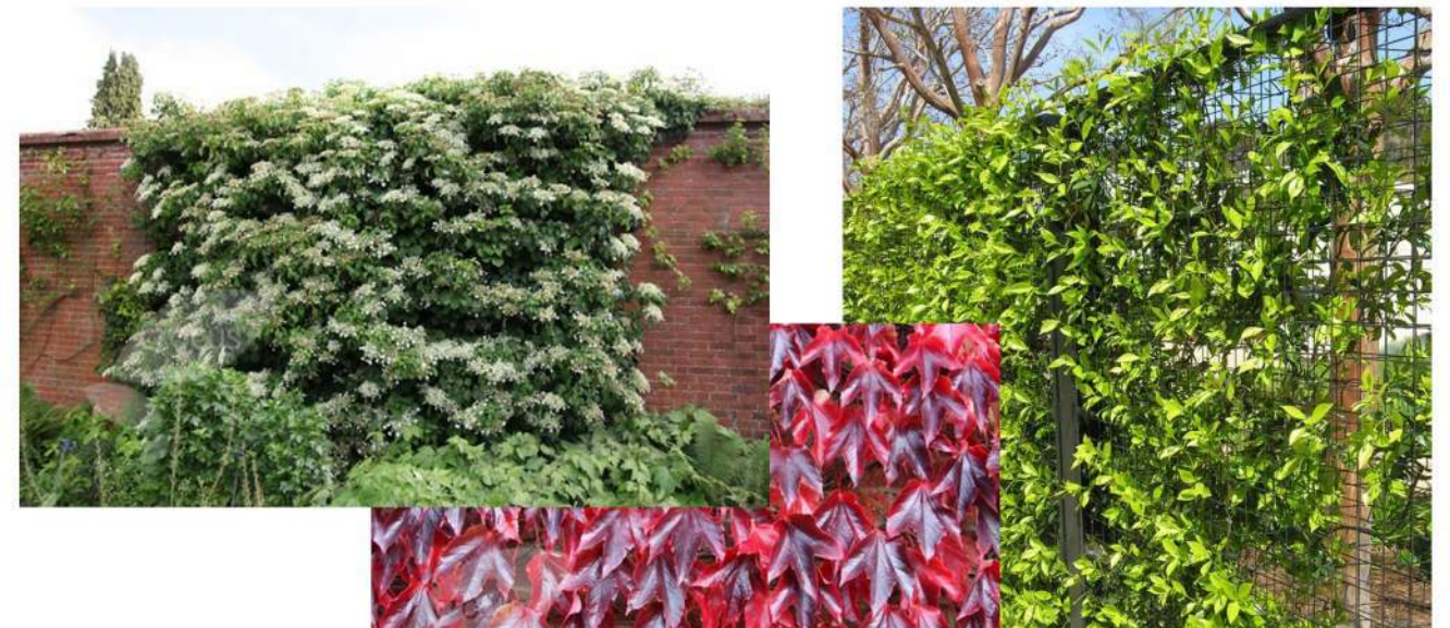
NORTH GREENROOF WALL AND HVAC SCREENING
